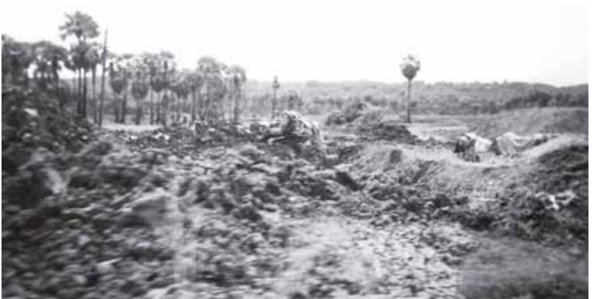
Railway constructors taking soil to build a railway bridge.
