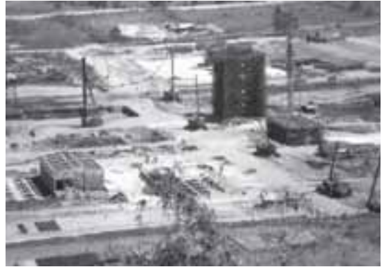
Iron factory under construction. Photo by PYO
