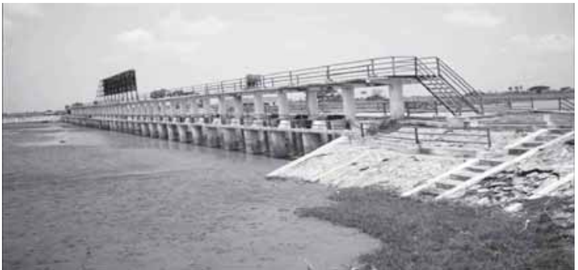
The upper and lower parts of the water gate.
