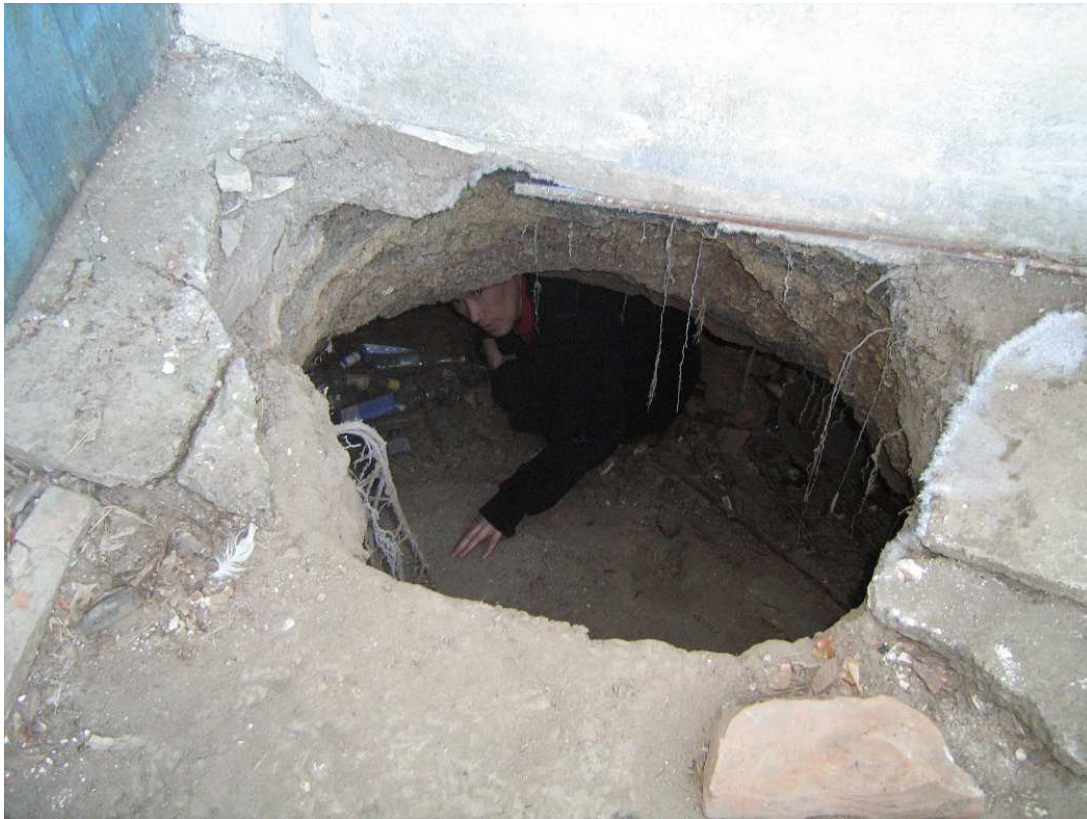
Sinkhole under Nagaisha Demesheva's house, the village Berezovka, January 2011
