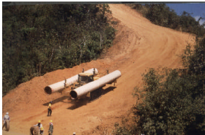
Yadana pipeline construction
