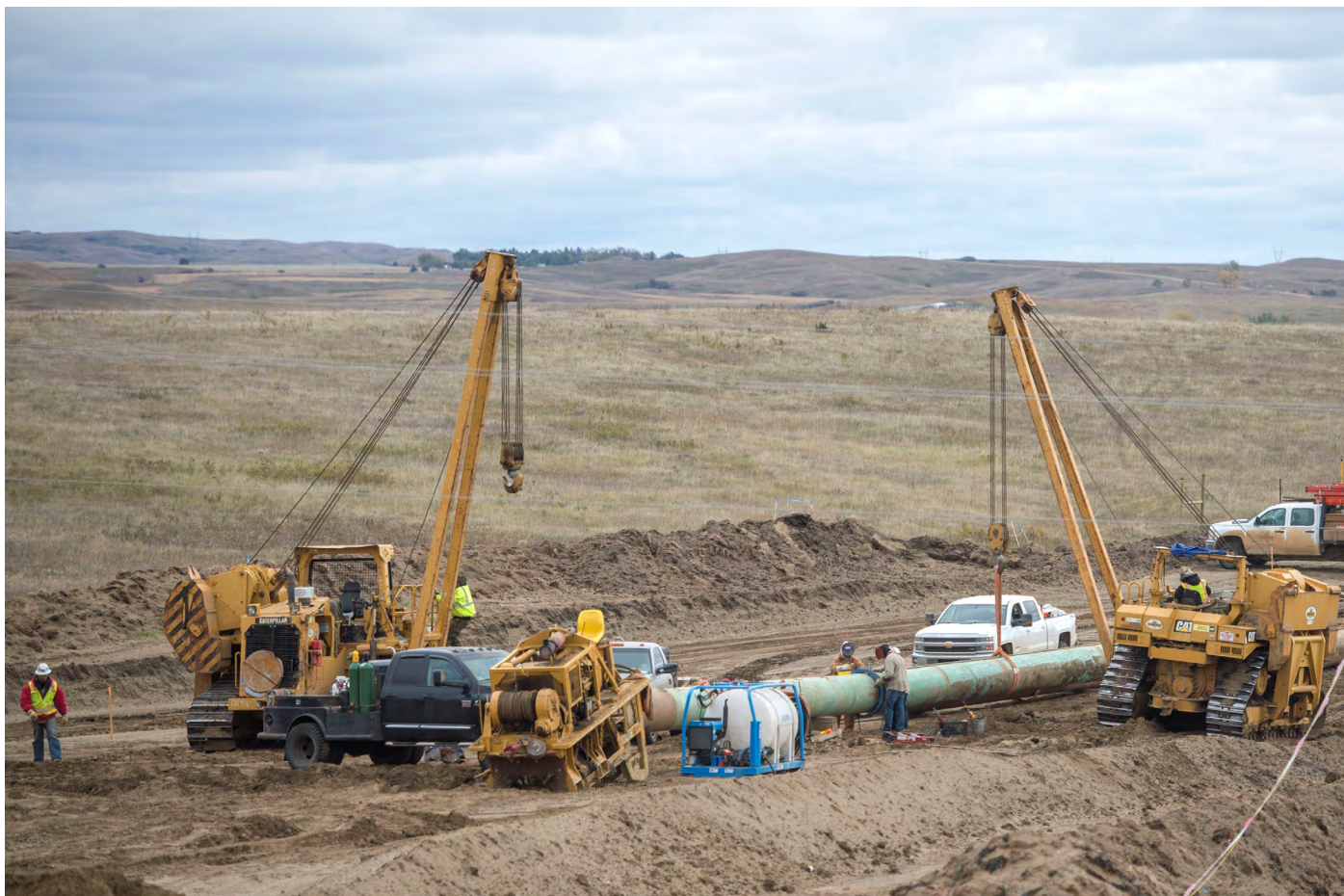
October 2016, construction resumes on the Dakota Access Pipeline south of Mandan, ND along State Road 6. © Photo by Cayla Nimmo
